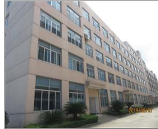
External photo(s) of the production unit(s) Production and warehouse combined building.JPG
